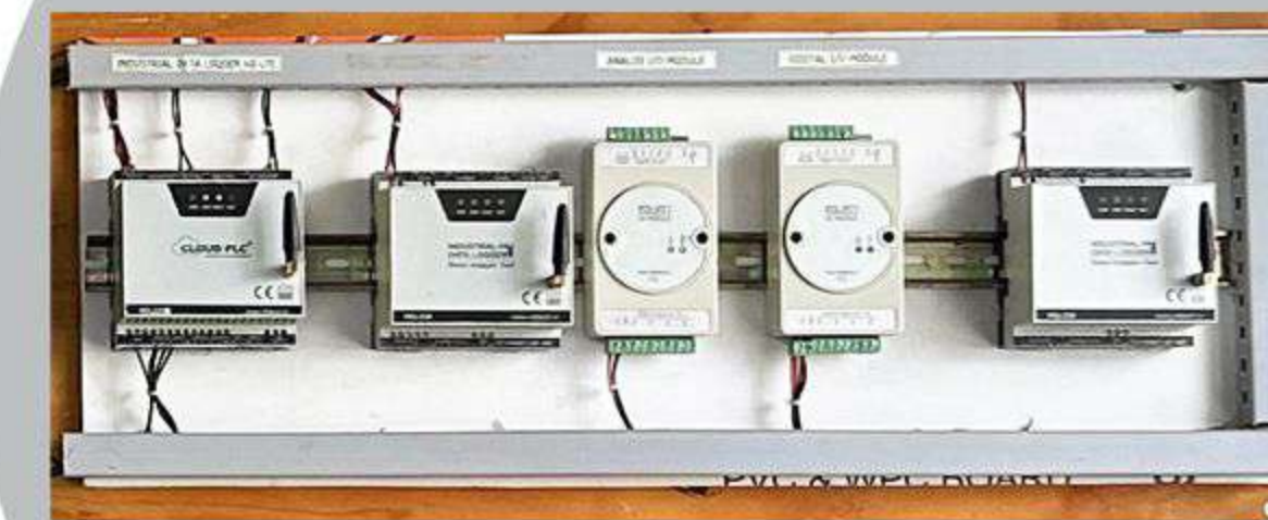
IO & Computing Modules Panel
